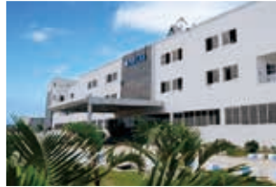
Rudrapur Plant (Green Building)
