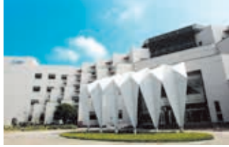
Tainan Plant (Diamond-rated Green Building)
