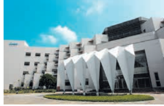
Tainan Plant (Diamond-rated Green Building)
