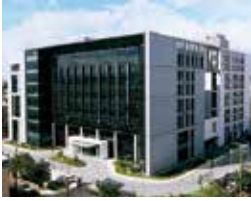
Taoyuan Technology Center (Green Building)
